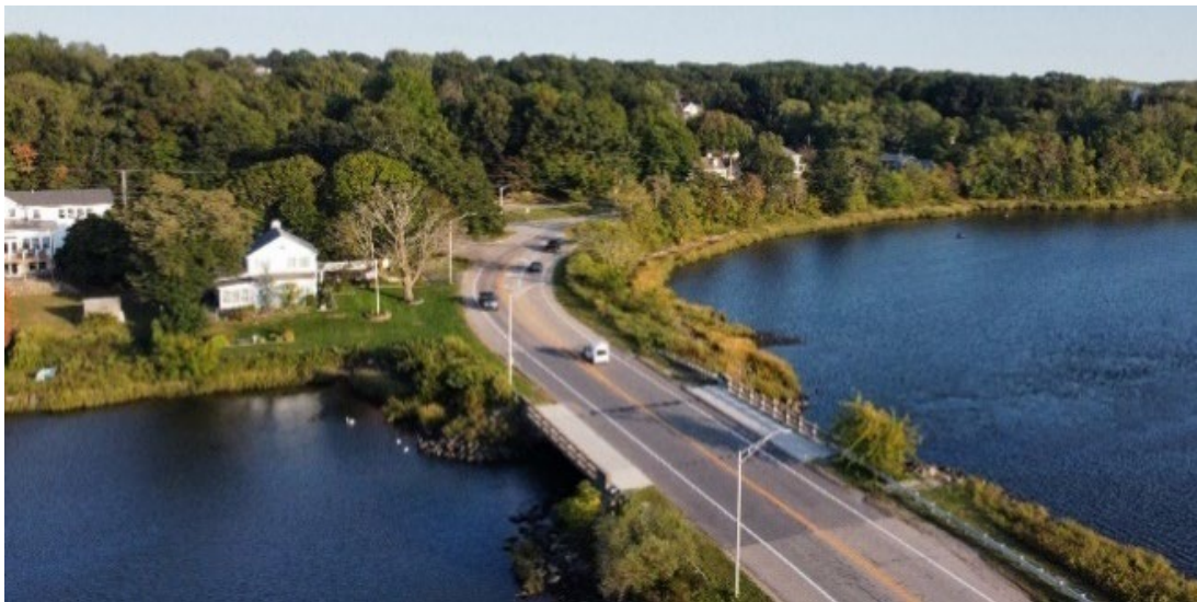
Figure 1-13. Bird's eye view looking east on Veterans Memorial Parkway, with bridge over Watchemoket Cove, East Providence, RI. Source: Elena Pascarella, Landscape Architect
