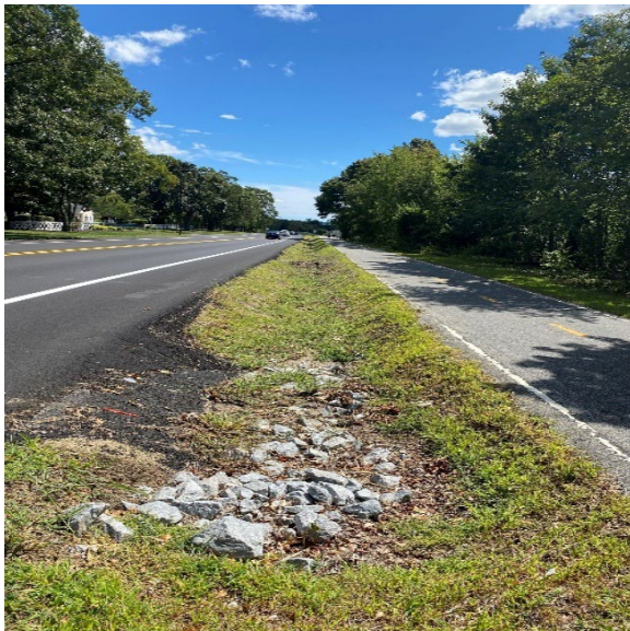
Figure 3-22 Appropriate for stormwater management. Drainage swale along Veterans Memorial Parkway and East Bay Bike Path. Source: Pam Sherrill
