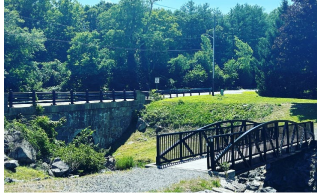
Figure 3-12. Multi-rail on Great Road in Lincoln, RI. Source: RIDOT
