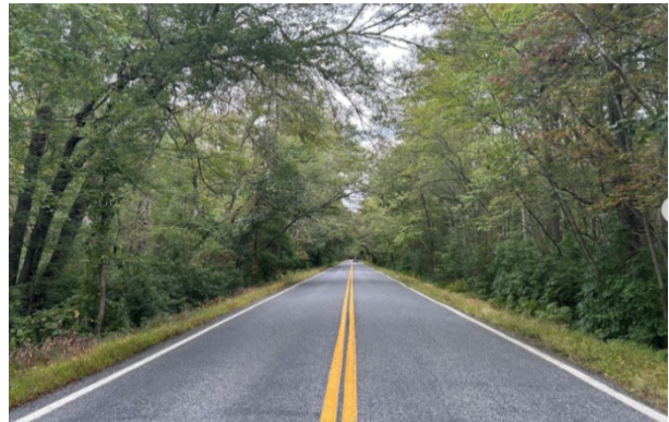
Figure 1-7. Ministerial Road, South Kingstown, RI. Source: RIDOT
