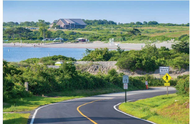
Figure 3-7. A view of Paradise Loop in Middletown, RI, that illustrates how scenic beauty is maintained without utility poles above ground. Source: Andrea Hansen, Newport This Week, August 2021
